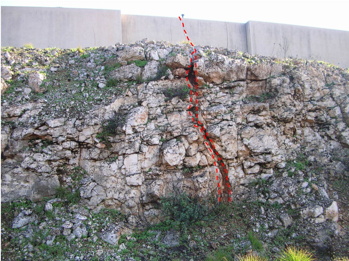
Fig. 6 : Karstified limestone beds. Notes inclined layering in landslide attitude (“traverpoggio”), one family of joint with narrow persistence and a likely fault plane. The hanging over wall is fault fracture plane affect, too (STOP 4)
